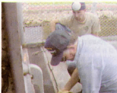
Newt & Ray working on expansion joint
