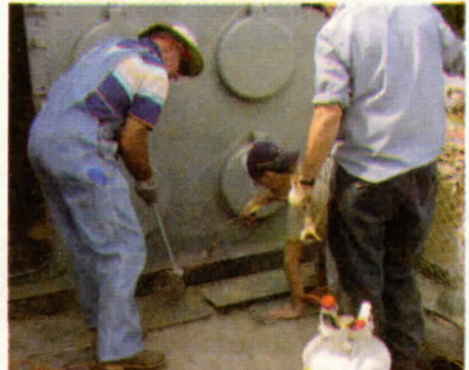
Repairing Expansion Joints
